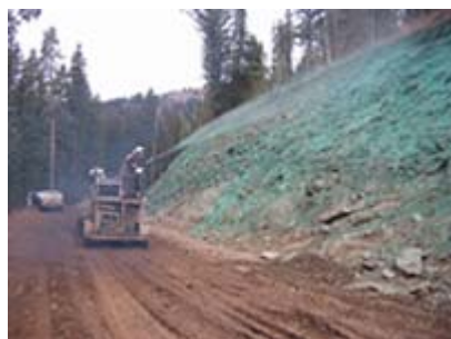
Hydro seeding pipeline diversion access road cut-off
